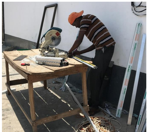
Construction of windows
