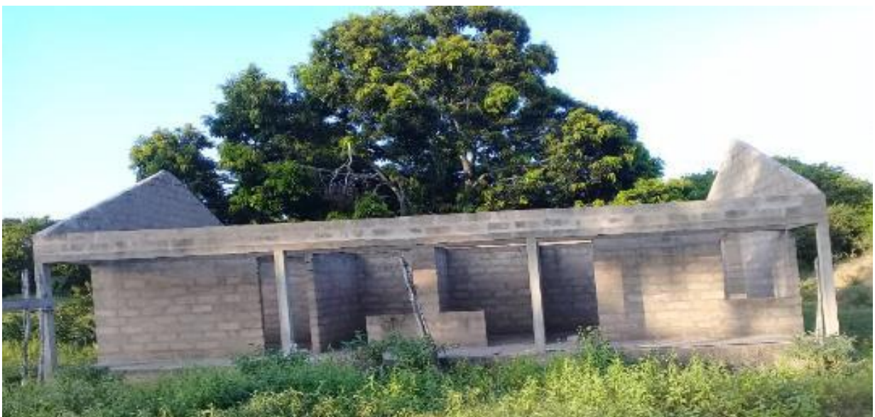
Start of the construction
